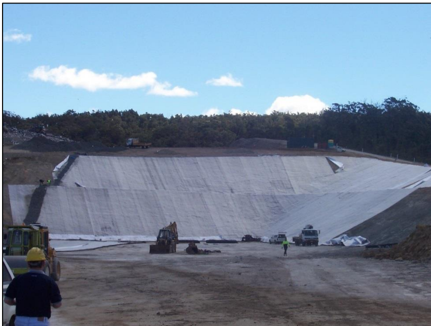
Geosynthetic Clay Liner being installed at a waste landfill site
